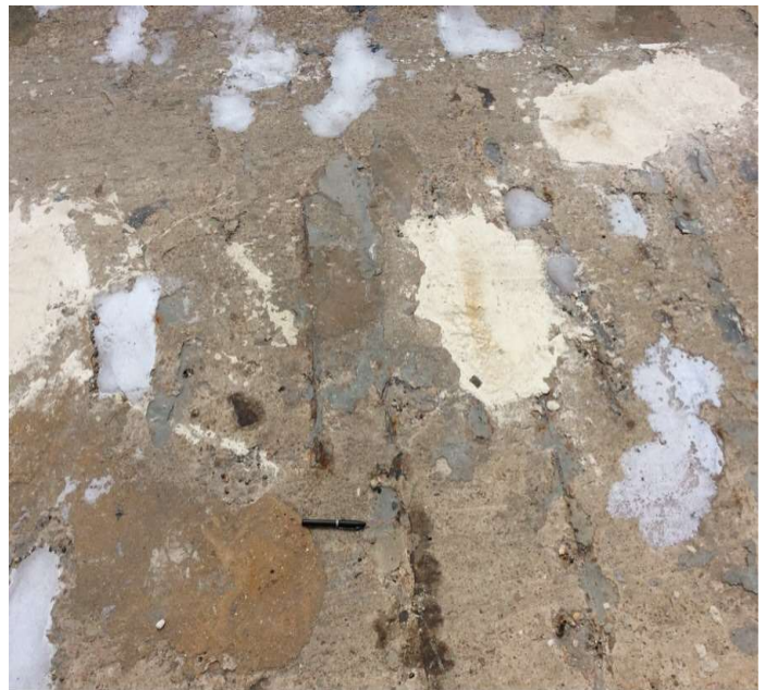
PHOTO 2 Description Deck spalls with rebar exposed
