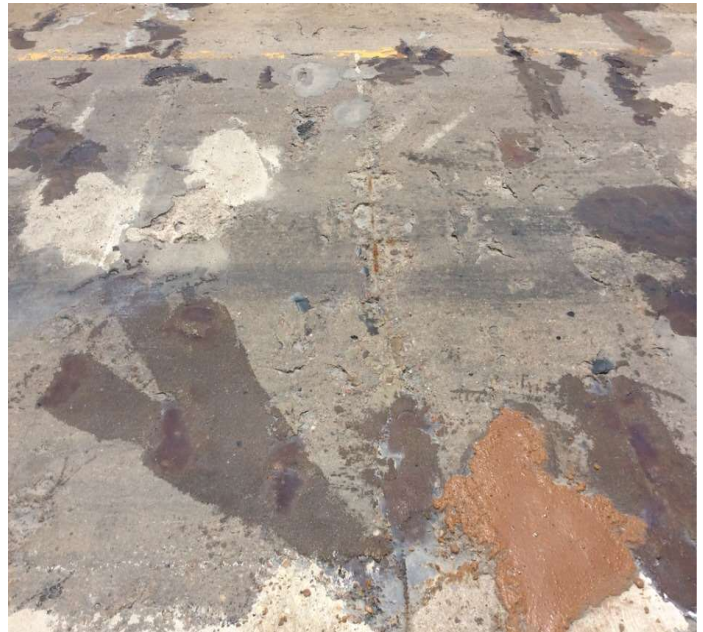
PHOTO 6 Description Deck spalls with rebar exposed
